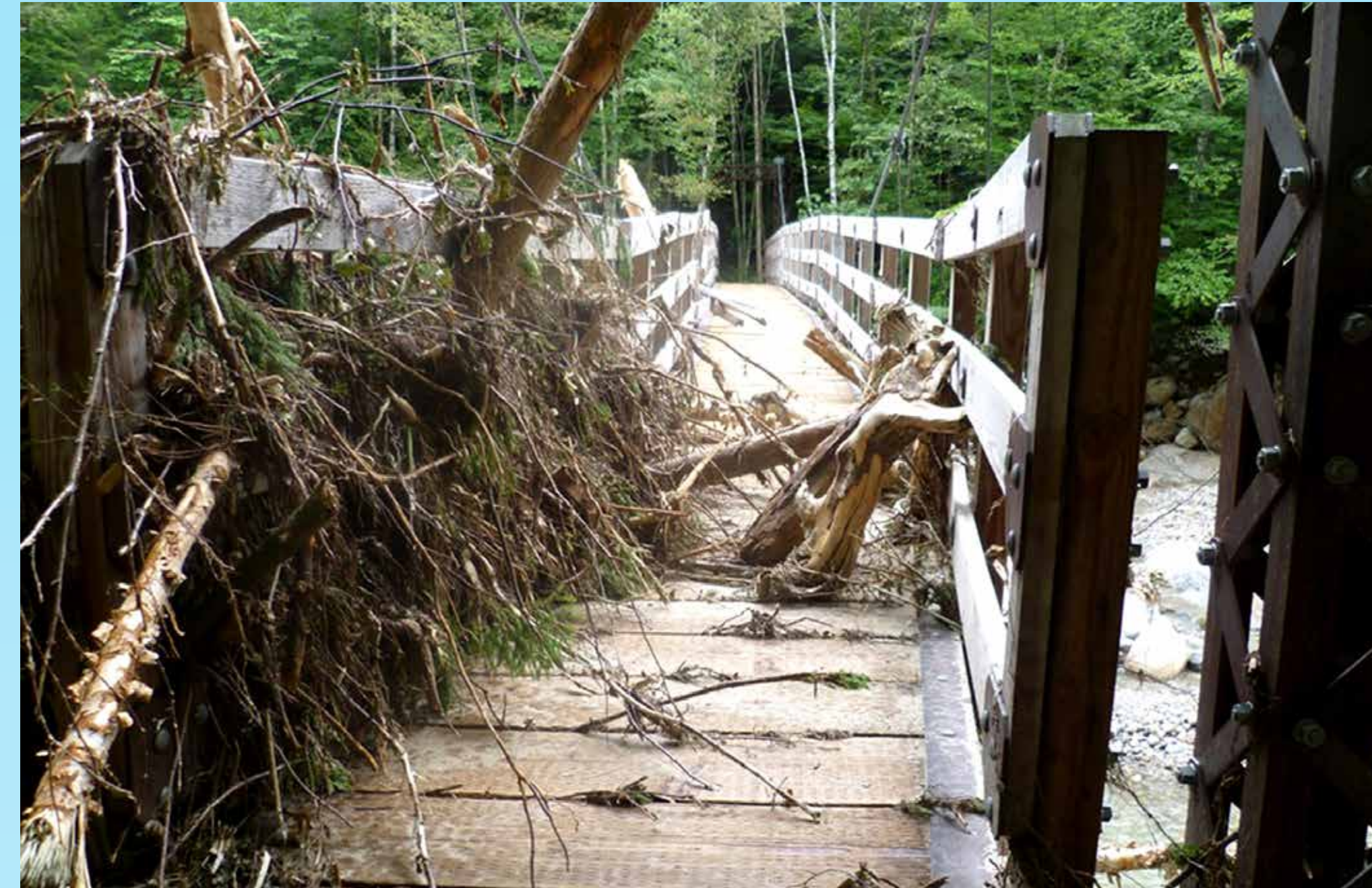
The Dry River, normally 35 feet below the bridge deck, left this debris after Irene.
