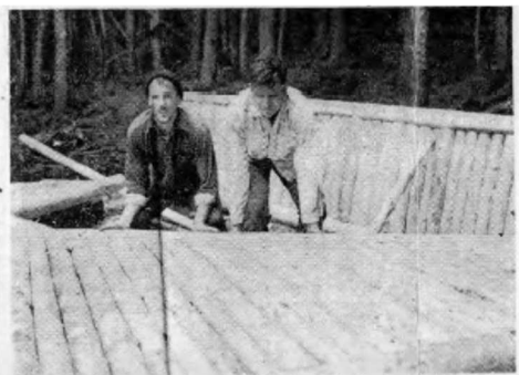
PREFABRICATION is the watchword with this trail crew. Having cut down trees and nailed one side of the shelter together, Lewis Gholston, Alabama, left, and Frank von Hippel, trail crew chief, get ready to lift it into place. When finished, this shelter will sleep 16 persons.
