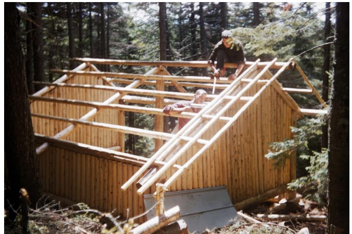
Lewis Gholston caulks and Warren Lightfoot sites the supports for the roofing (courtesy of RB or FvH).
